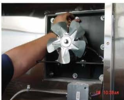
Step 5 - Remove Nuts, Lock Washers & Washers.
