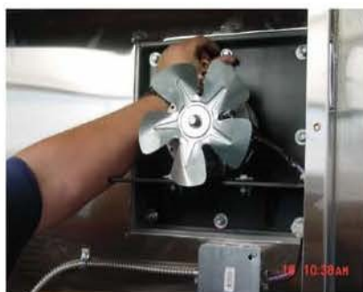
Step 5 - Remove Nuts, Lock Washers & Washers.
