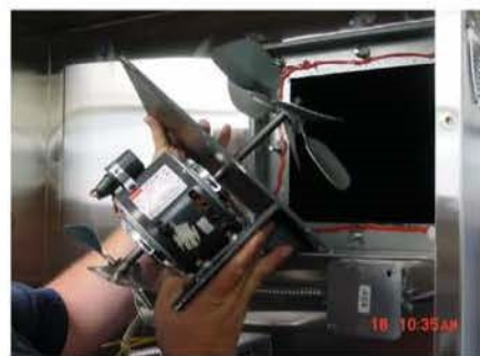
Step 7 - Slowly Remove the Convection Fan Assembly(s).
